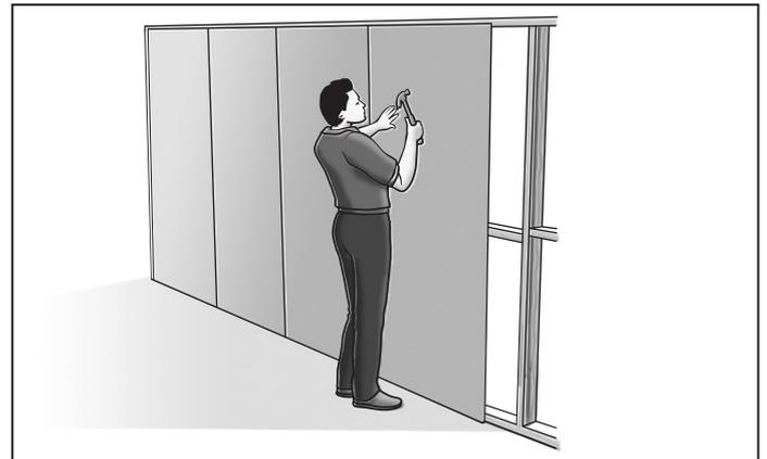
FIGURE 5 SHEET INSTALLATION
